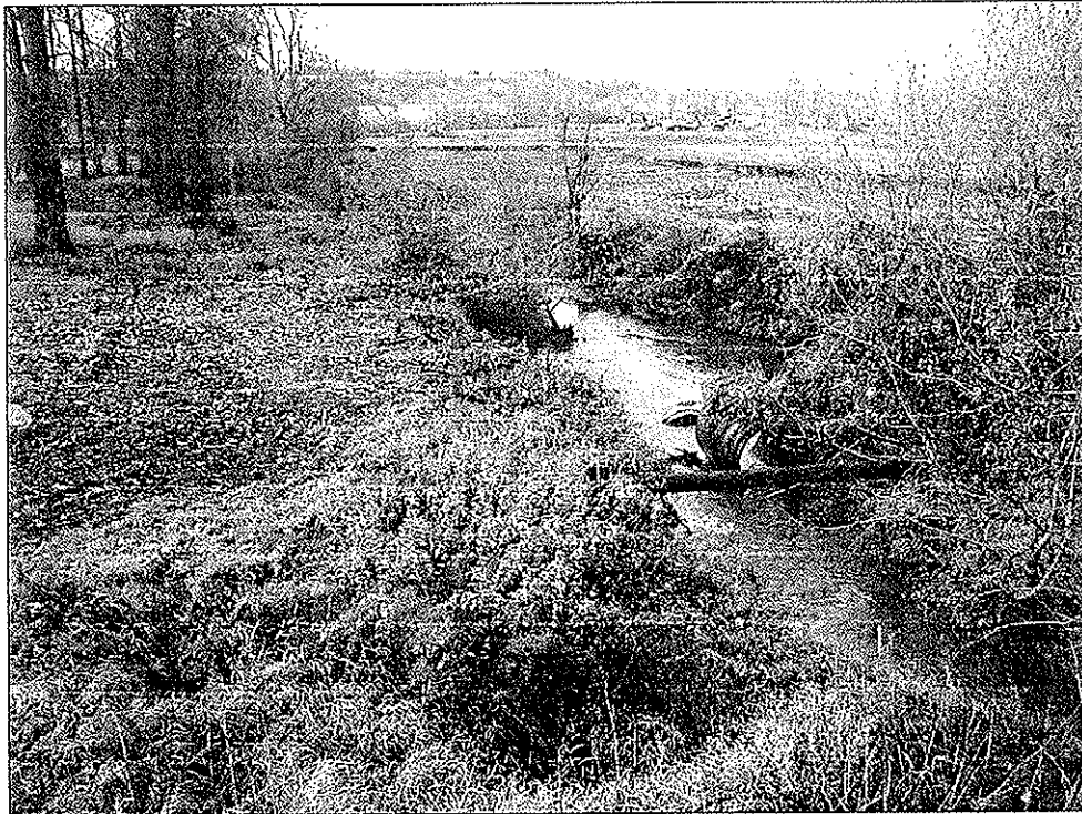
Above: photograph looking west from railroad tracks at Salmon Creek. Note old culvert sections and debris in channel.
